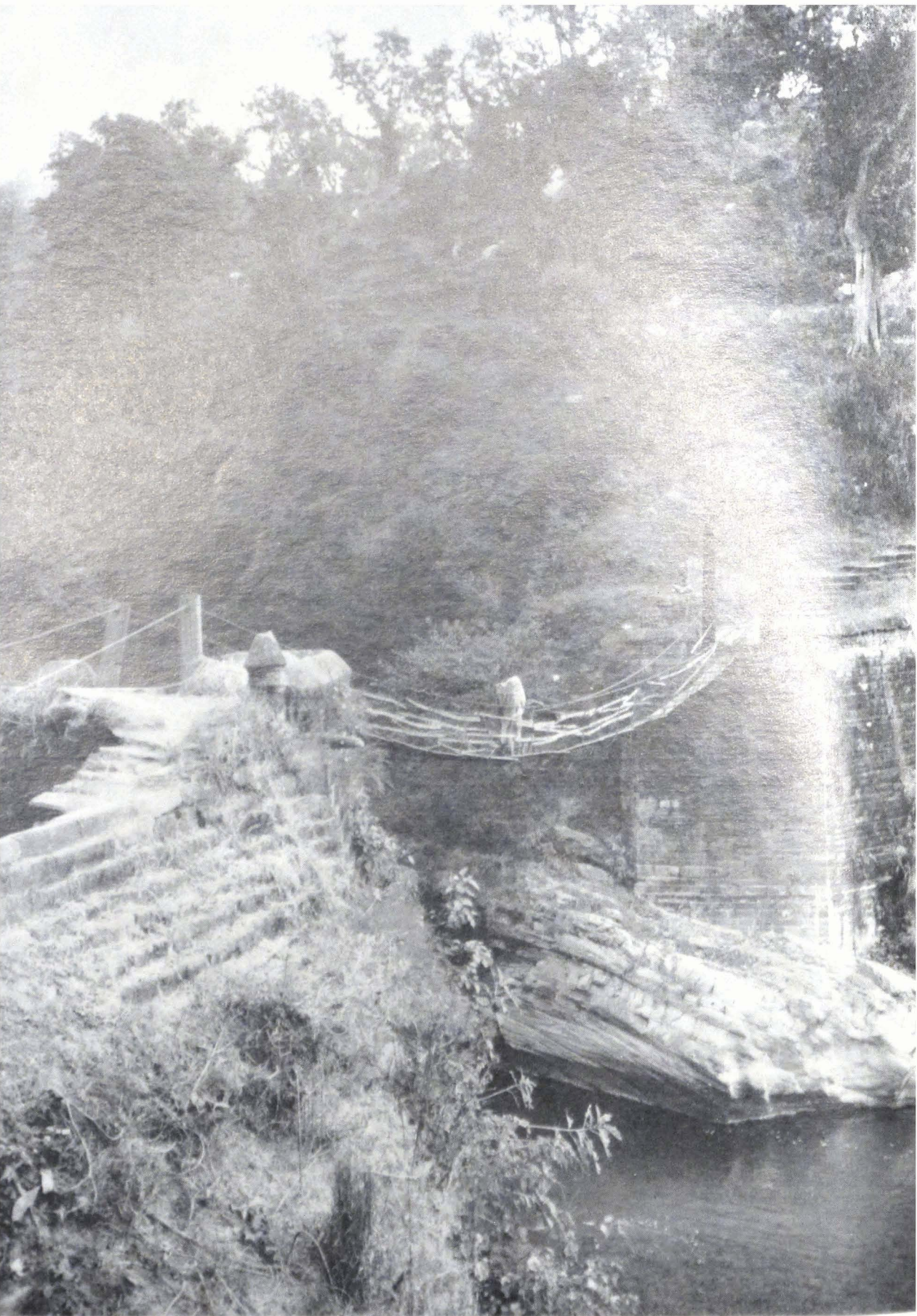
15. Gurkha district: bridge in typical state of disrepair.
